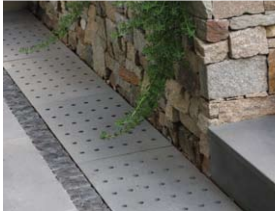
Bluestone [Custom Drainage Grate] [08]
